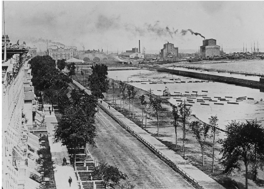
FIGURE 4: LAKE PARK “ROWHOUSES ALONG MICHIGAN AVENUE OVERLOOKING RIVER AND FACTORIES, LOOKING NORTH FROM HARRISON STREET CIRCA 1865” 51
