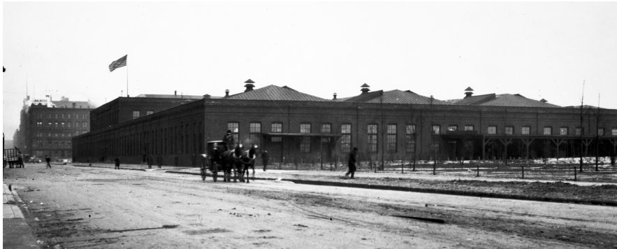
FIGURE 16: TEMPORARY POST OFFICE IN GRANT PARK AT WASHINGTON STREET CIRCA 1900 531
