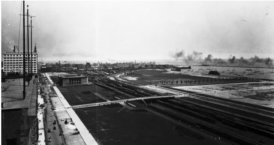
FIGURE 8: “MICHIGAN AVENUE. BIRD’S EYE VIEW NORTH FROM HARRISON STREET 1913,” SHOWING LANDFILL AND THE ART INSTITUTE AS THE ONLY BUILDING IN GRANT PARK 104
